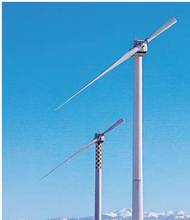
Figure 1.14 - Single-blade with counterweight turbine
