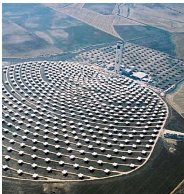
Figure B.8 – Central receiver plant
