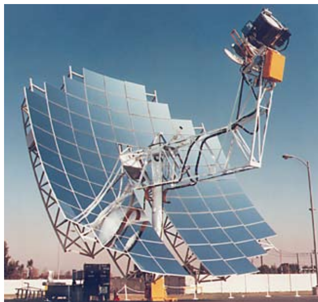
Figure B.6 - Parabolic dish plant
