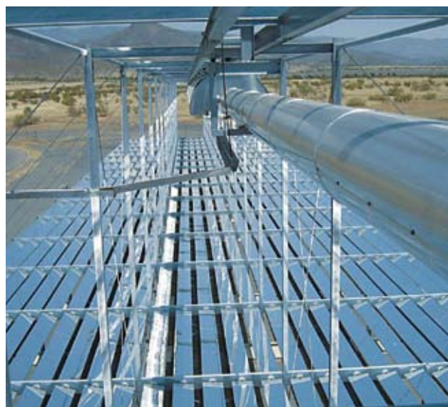
Figure B.7 - Linear Fresnel concentrator plant
