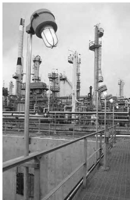
Enclosed and gasketed CHAMP® luminaires providing walkway lighting
