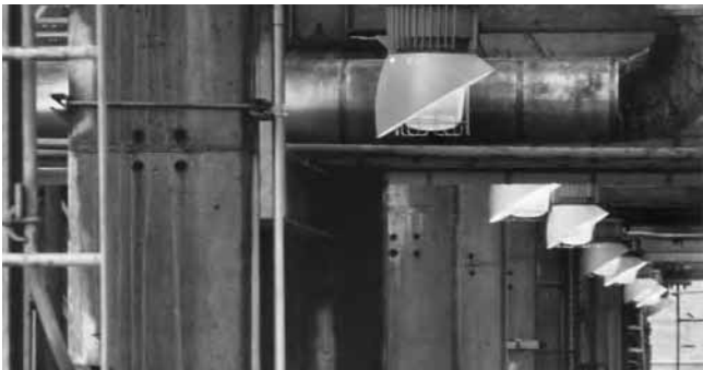
Class II luminaires allow lights to be placed where they are needed most, without fear of causing a fire from sparks or overheating.
