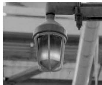
VAPORGARD™ luminaires in oil refinery
