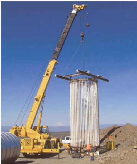
Fig. 2: Lowering assembled bolt cage.
