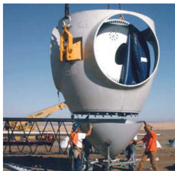
Fig. 4: Assembly of nacelle in marshalling yard.
