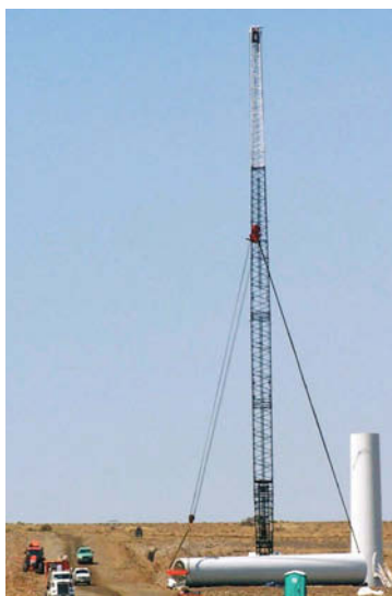
Fig. 5: Erecting tower base with wheel-mounted crane.
